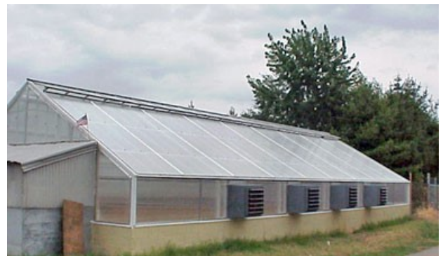
After: Re-glazed greenhouse
