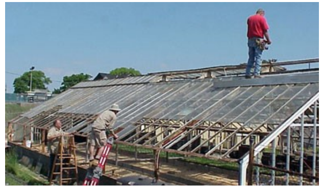
In progress: Removal of glass
