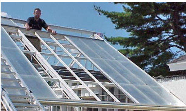
Re-glazing in progress
